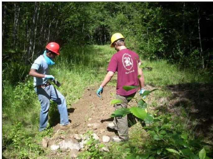
Building tread width in Sleepy Hollow
